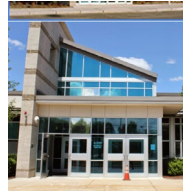
GLFHC Greater Lawrence Technical School
